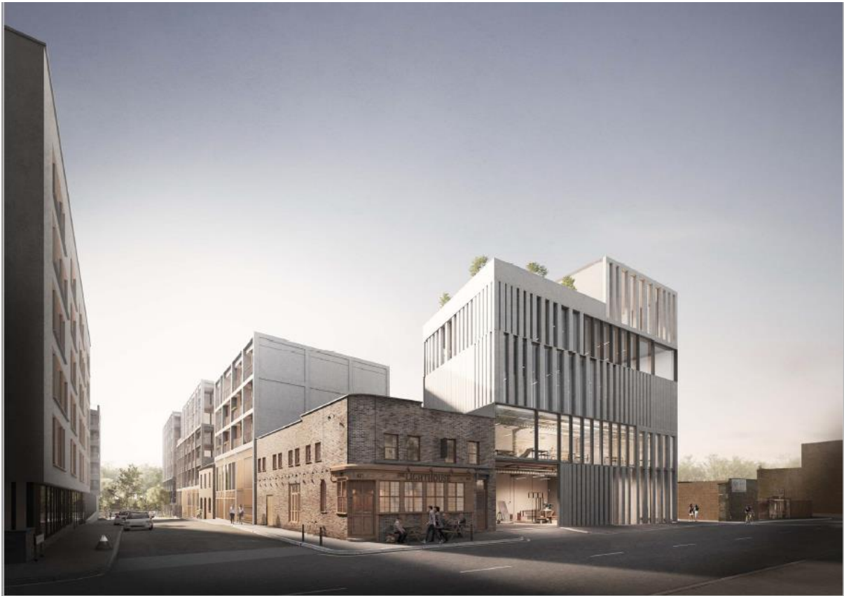
View from Wick Lane
